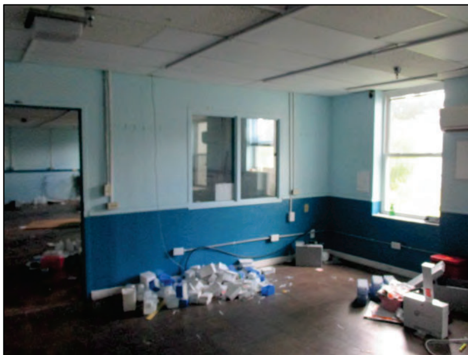
TYPICAL INTERIOR VIEW OF MAIN HOSPITAL FACILITY
