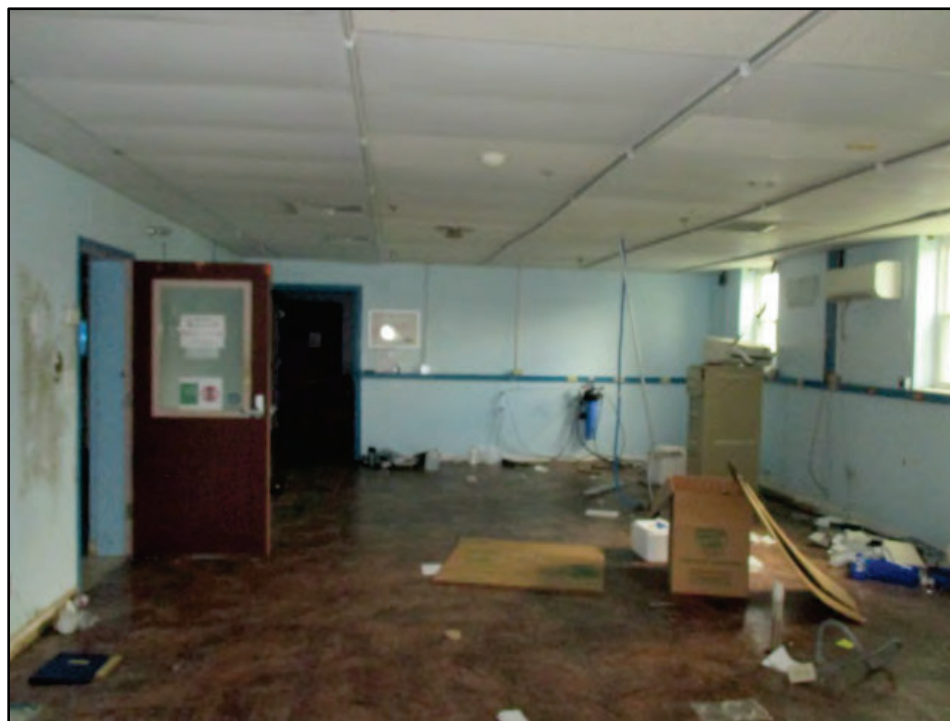
TYPICAL INTERIOR VIEW OF MAIN HOSPITAL FACILITY
