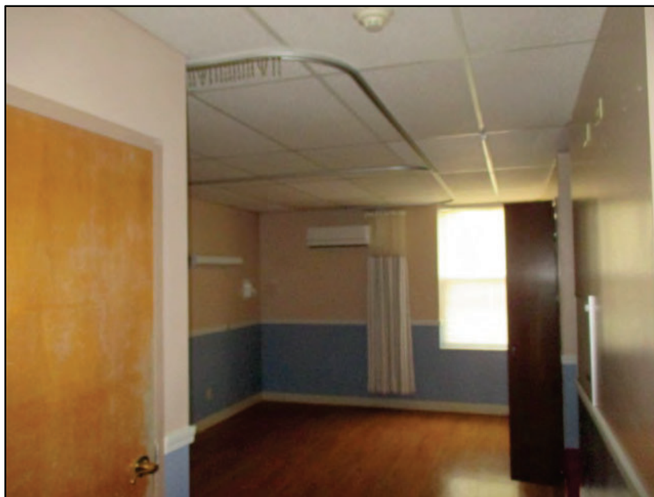
TYPICAL INTERIOR VIEW OF MAIN HOSPITAL FACILITY
