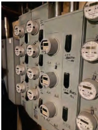
Separate Electric Meters
