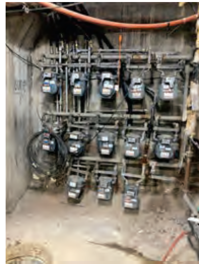
Separate Gas Meters
