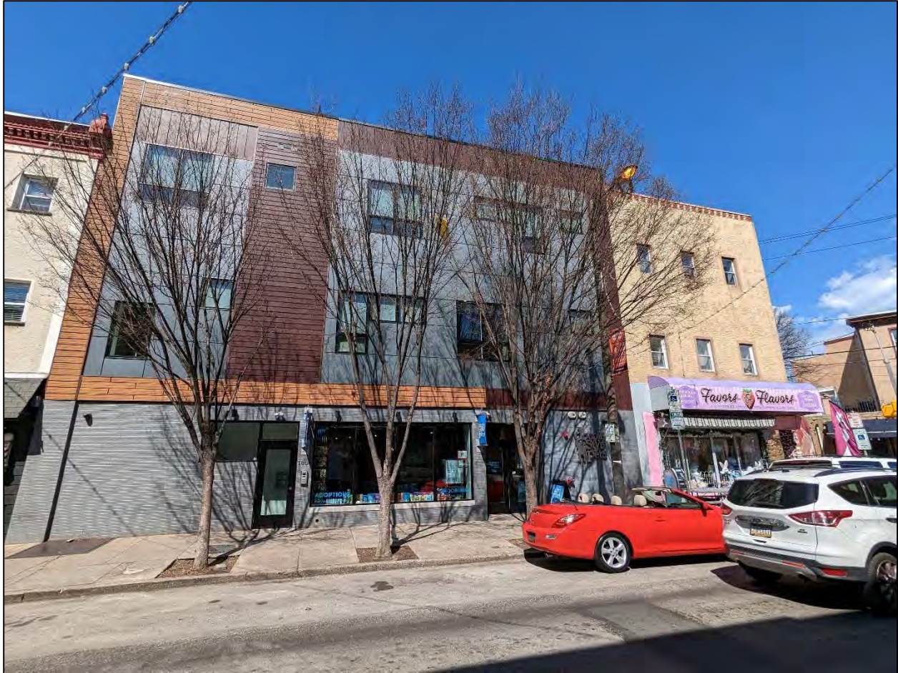
New construction mixed use along East Passyunk Avenue
