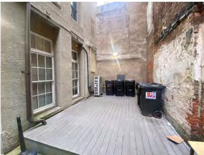
REAR BUILDING VIEW
