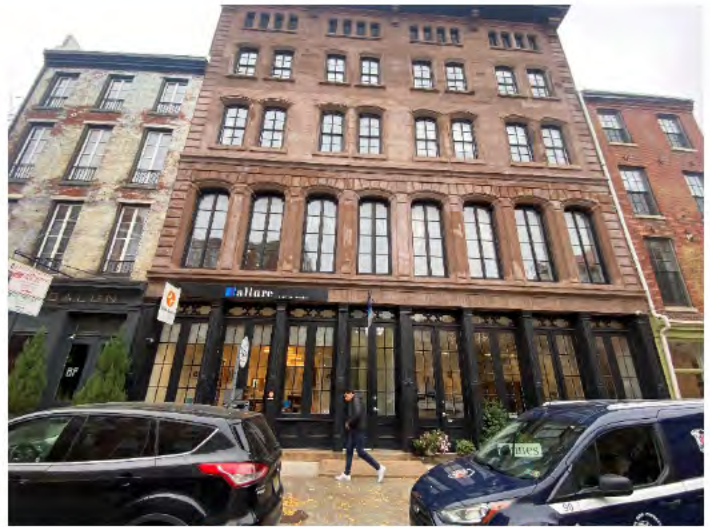
FRONT BUILDING VIEW
