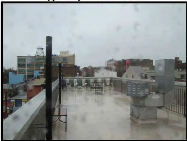
View of Roof Deck
