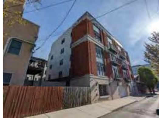
Subject viewed northeast
