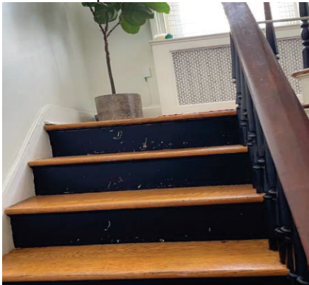
Bi-Level Unit Stairwell
