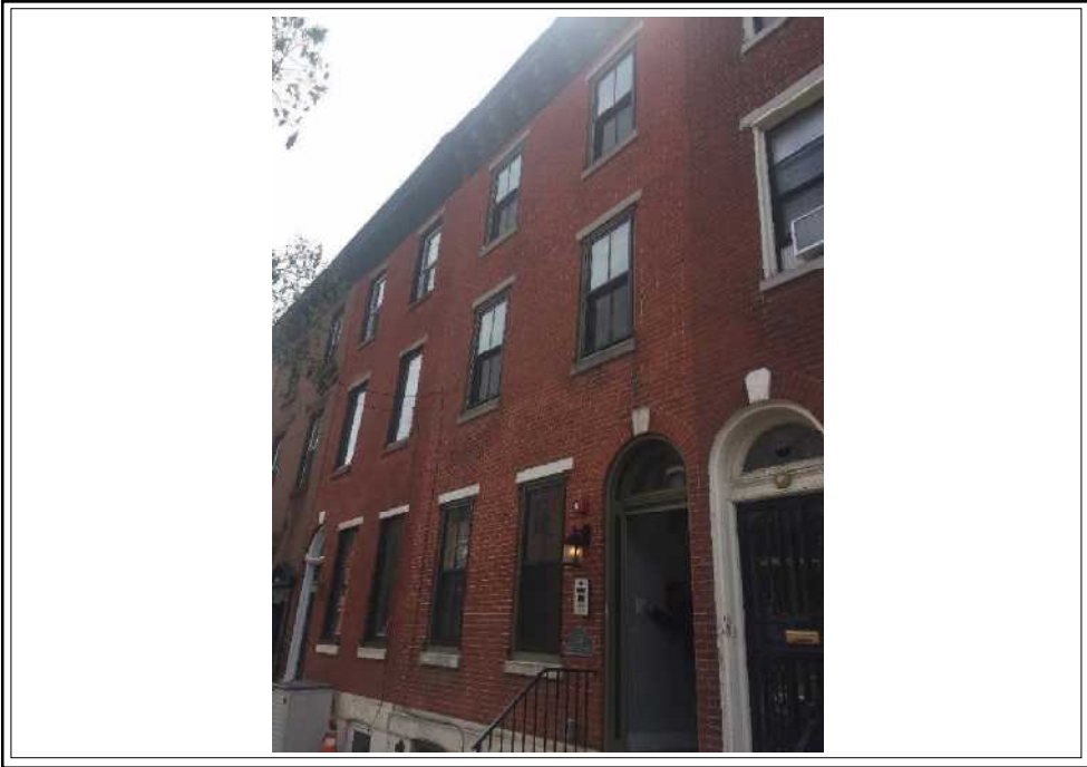
FRONT VIEW OF SUBJECT PROPERTY
