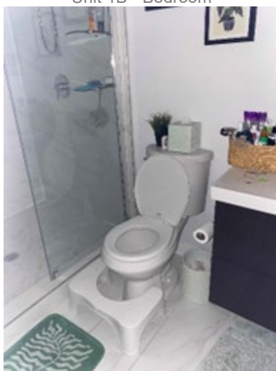
Unit 1B - Restroom
