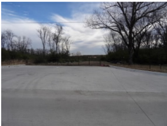
Street View: Curb Cut on Old Decatur Road
